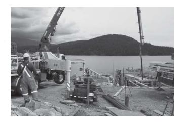
slides down the pipe, it develops a vacuum which greatly expands the air bubbles; and when they hit an elbow in the boom or a horizontal surface, the bubbles collapse. Naturally, the transition from several hundred MPa of pressure in the line to a near vacuum condition may make matters worse. Most field experience suggests that air loss is greatest with rich, flowable mixes which slide down easier; however, air loss has also been experienced with 300kg/m³.
