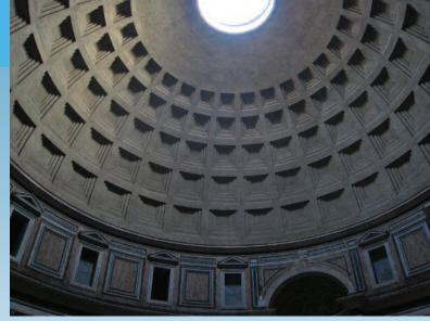
**The Pantheon in Rome** is one of the world's most remarkable interior spaces, and, after nearly two thousand years, it is still the largest unreinforced concrete dome on earth.
