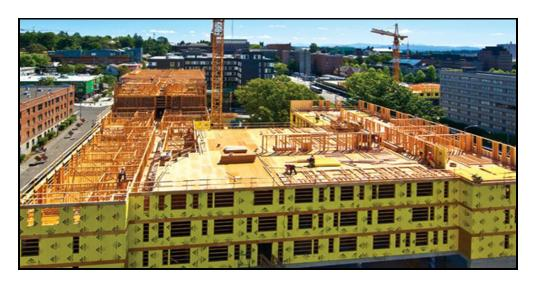
For this project in the Pacific Northwest, protecting wood from moisture was a priority. The yellow exterior sheathing is mold-resistant drywall. Although not shown in this photo measures to protect moisture ingress from rain, during construction, both from above and from wind-driven rain through the openings are equally important. Mold-resistant drywall is a 'post-construction' strategy.'
