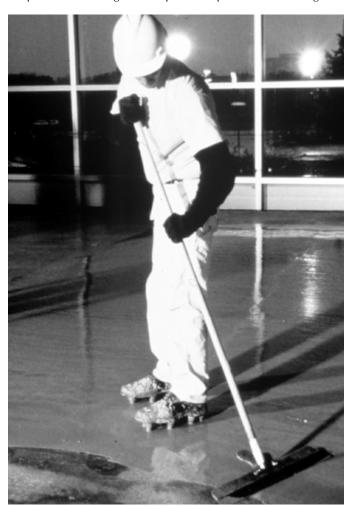
Figure 13. Self-leveling toppings can be used to restore the floor surface on an otherwise sound slab. Underlayments usually require a floor covering material such as tile or carpet. (69682)
