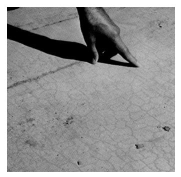
Figure 4. Crazing is a network of fine surface cracks. (4099)
