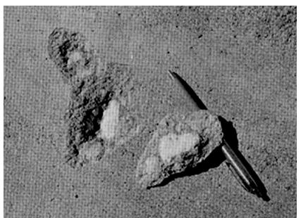
Figure 8. A popout is a small fragment of concrete surface that has broken away due to internal pressure, leaving a shallow, typically conical, depression. (0113)
