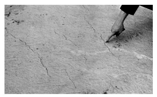
Figure 2. Plastic-shrinkage cracks caused by rapid loss of mix water while the concrete is still plastic. (1311)
