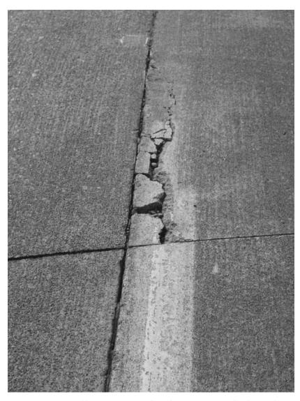
Figure 11. A typical location for a spall is along a joint, usually the result of the joint functioning improperly. (67216)
